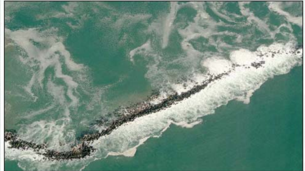
Pt. Judith Breakwater Harbor of Refuge
