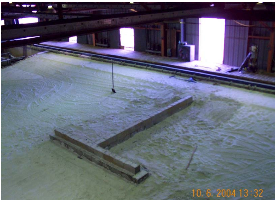
Figure 112. Third layer concrete block T-groin core.
