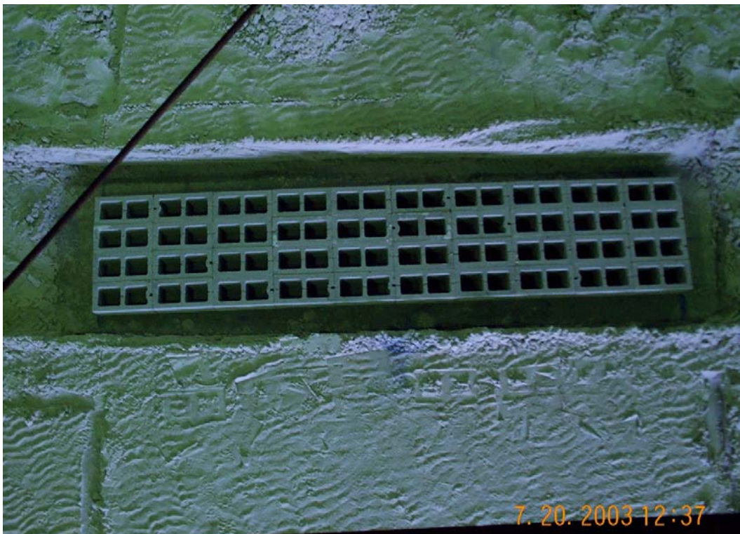
Figure 27. Concrete block breakwater foundation and core.
