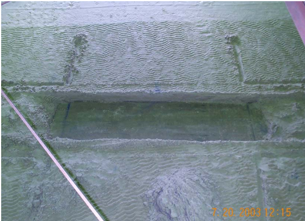
Figure 26. Excavated sand beach for breakwater construction.
