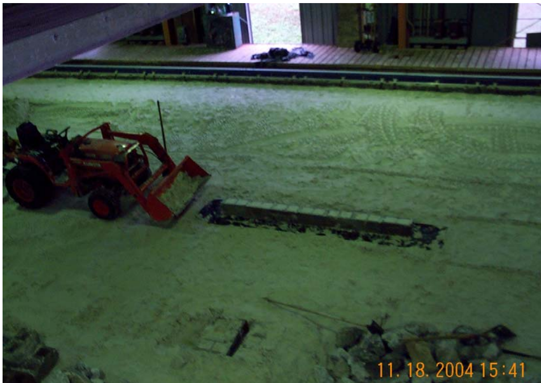
Figure 143. Nearshore breakwater with filter cloth covering foundation layer and second row of sand-filled blocks.
