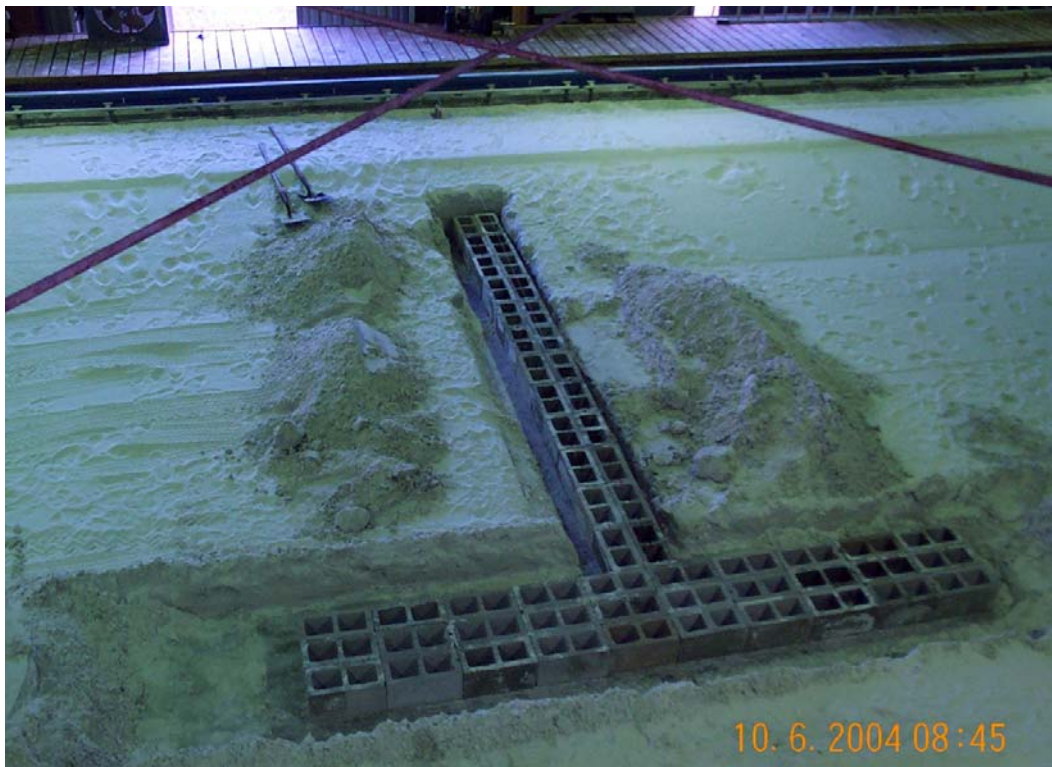
Figure 109. T-groin foundation and core.
