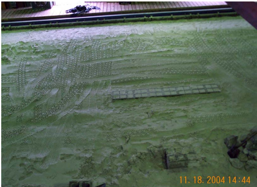
Figure 142. Breakwater foundation and core.
