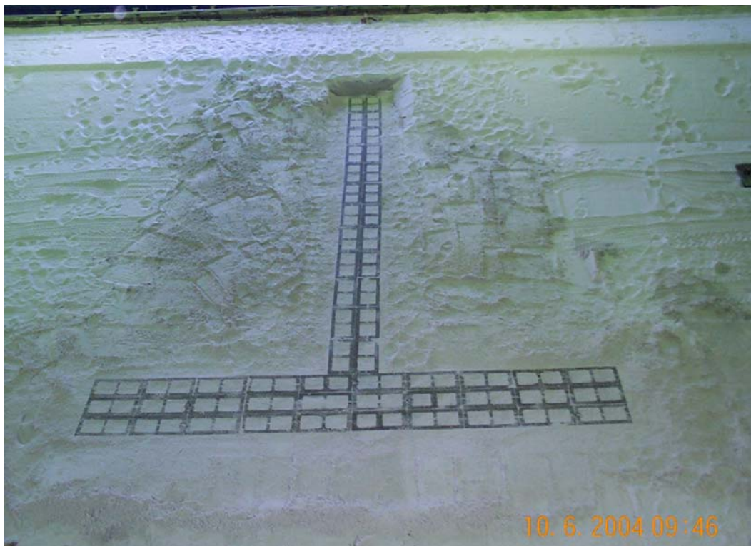
Figure 110. T-groin foundation backfilled with sand.
