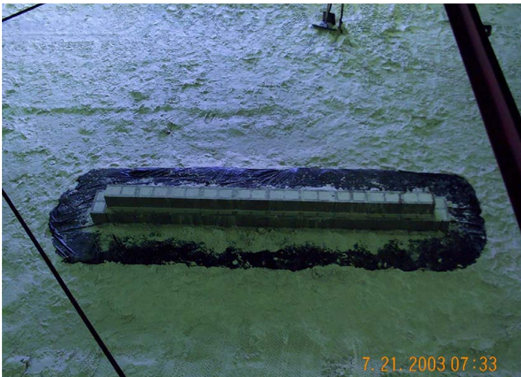
Figure 29. Third layer concrete block breakwater core.
