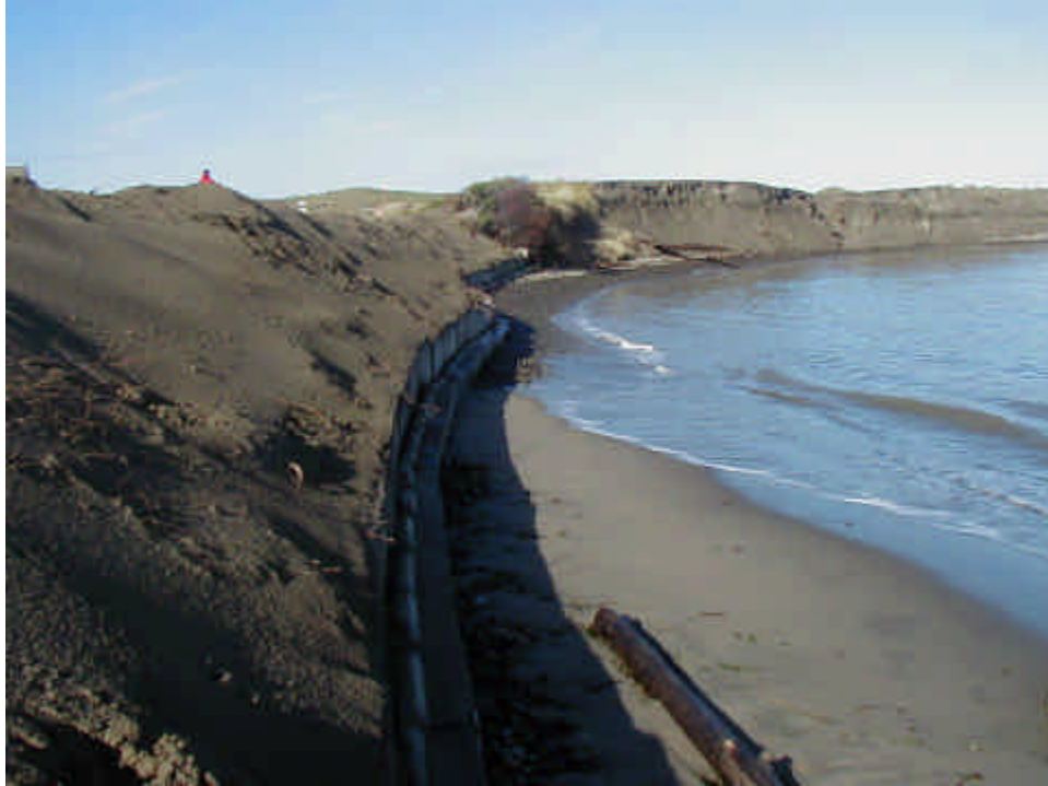
Figure 2-11. Temporary erosion protection, 23 October 2003
